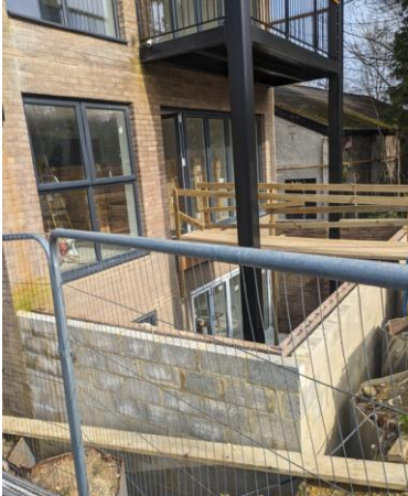
Figure 36 – Rear of 58 Whytecliffe Road South showing balcony/lightwell relationship to windows.
