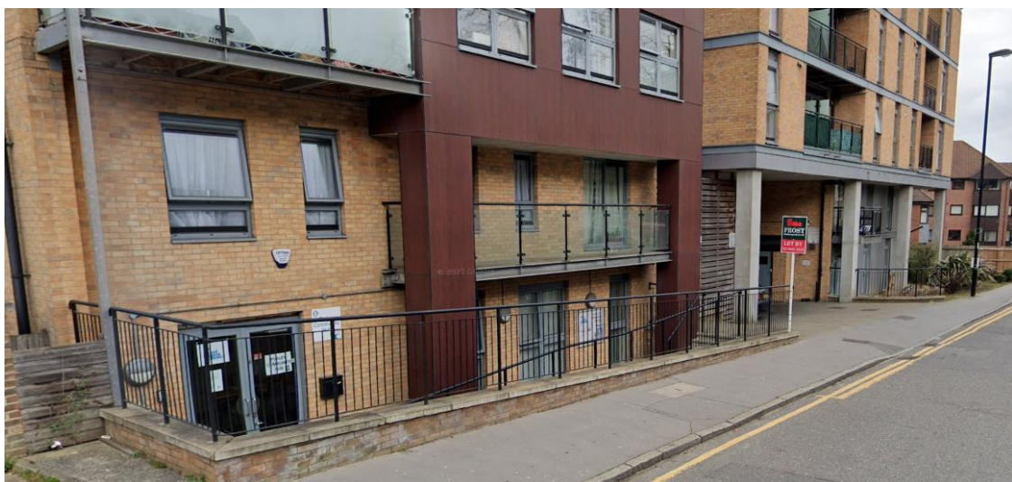
Figure 30 – Photo of lower two floors of Whytecliffe Road South
