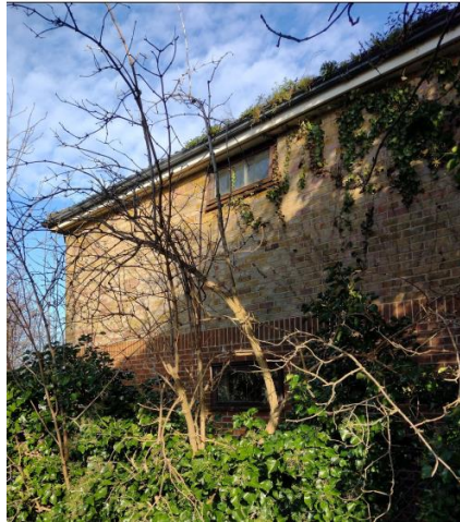
Figure 37 – Window on side elevation of 37 to 41 Redbarn Close
