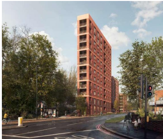
Figure 18 - CGI of granted planning permission 20/06224/FUL taken from junction of Foxley Land, Purley Way and Pampisford Road junction.
